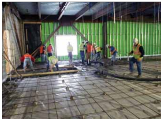
Left photo: Contractor crews pour the concrete slab in the Wellness area. Right photo: Workers finish the slab later that afternoon.
