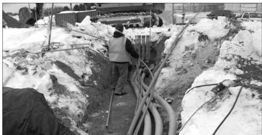
Heavy duty wiring connecting the new building with the transformer vault..
