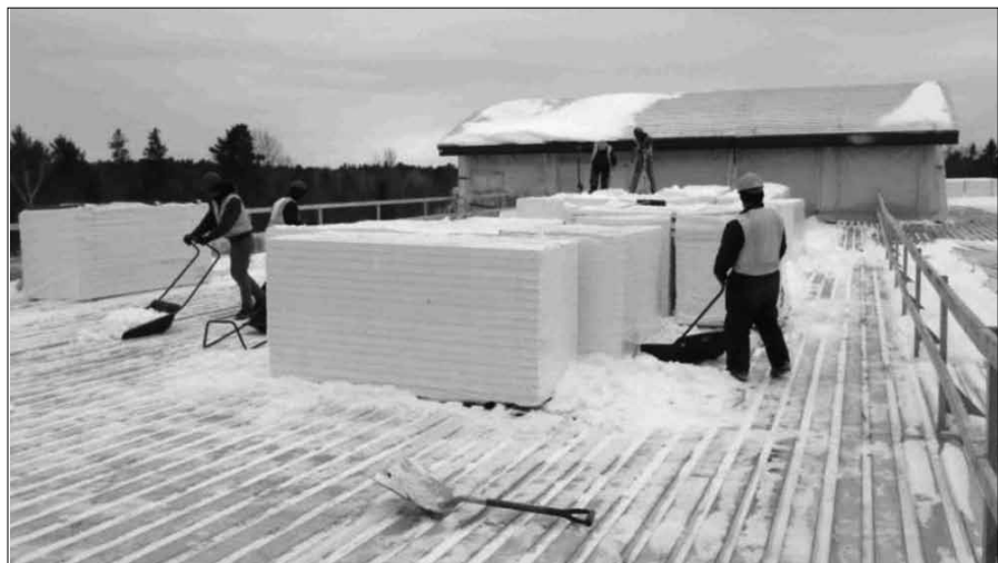
Workers shovel snow off the Classroom Wing roof.
