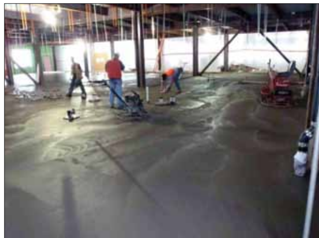
Left photo: Contractor crews pour the concrete slab in the Wellness area. Right photo: Workers finish the slab later that afternoon.
