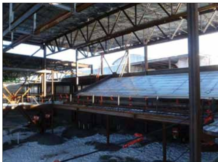
Steel work for the Performing Arts Center balcony.
